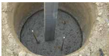
Feet to be fixed with concrete
