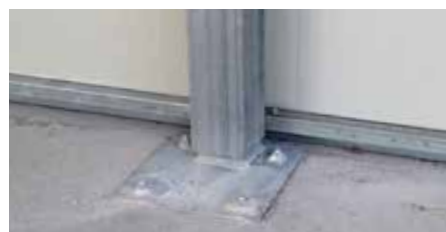
Feet with chemical dowels
